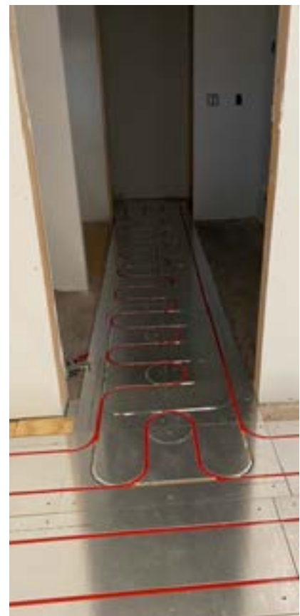
Note the creative tubing layout designed to route tubing from the room down this narrow hallway.
