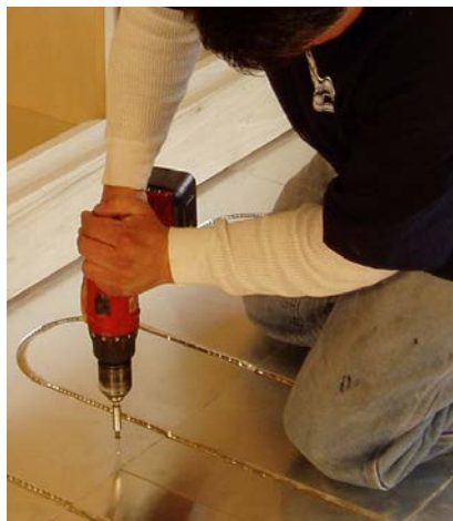
SCREWING Thermalboard™ BOARDS
